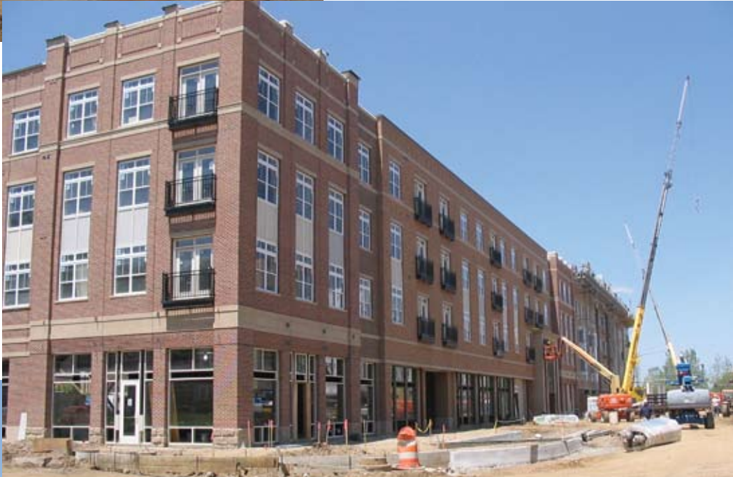
Views of Eddy Street Commons construction throughout the past year.
